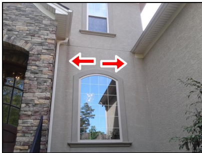
Front exterior wall
