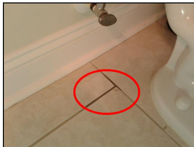
Rear bath under toilet
