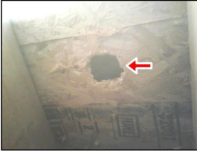
Left rear attic area
