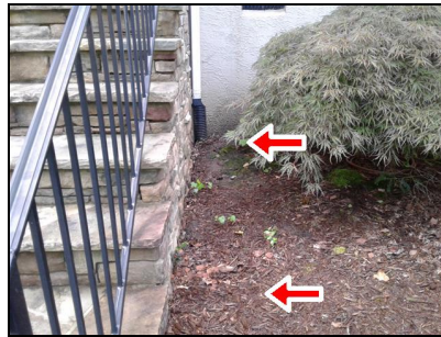
Front plant bed
