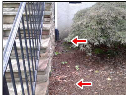
Front plant bed
