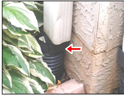
Disconnected downspout
