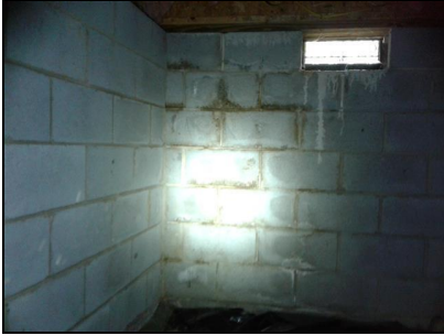
Foundation wall under dining room
