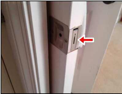
Rear hall bath pocket door frame
