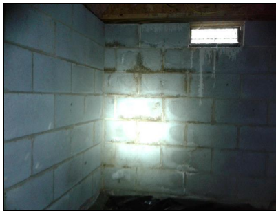
Foundation wall under dining room
