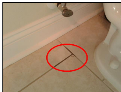
Rear bath under toilet
