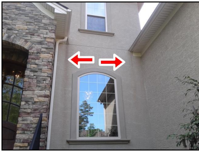
Front exterior wall
