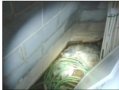
Left front crawlspace area
