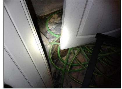
Left front crawlspace area
