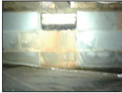
Rear foundation wall
