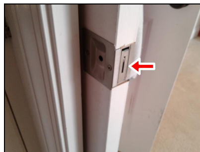
Rear hall bath pocket door frame
