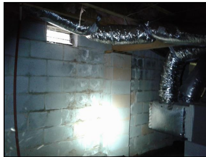
Foundation wall under dining room
