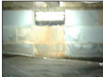
Rear foundation wall
