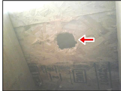
Left rear attic area
