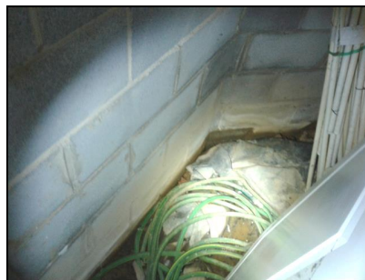
Left front crawlspace area
