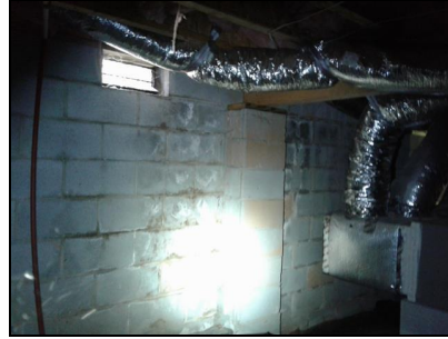
Foundation wall under dining room
