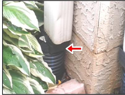
Disconnected downspout
