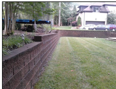
Rear stone retaining wall
