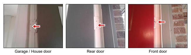
**2.4** Observed that the rear door rubs / hits the frame. Condition is conducive to further damages. Evaluation / Correction by a qualified handyman contractor is recommended for this entire condition.
