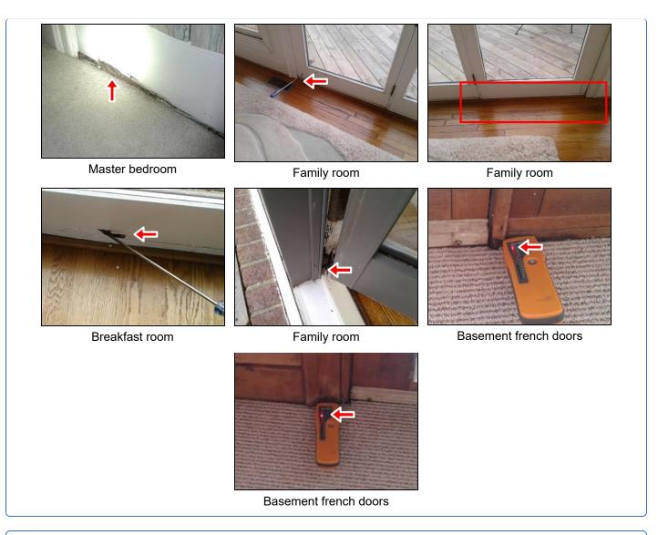
**2.4** Observed missing hinges screws at several exterior doors (See photos for locations) Condition is conducive to door sagging, rubbing over a period of time. Evaluation / Correction by a qualified handyman contractor is recommended for this entire condition.
